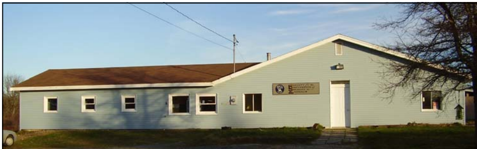
The Yarmouth SPCA Shelter
